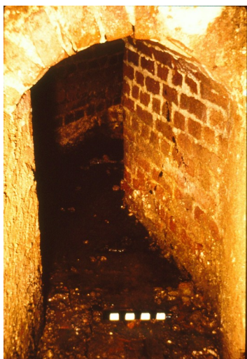
Vaulted drain entry
